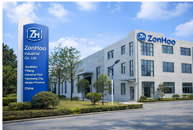
ZonHoo Manufacturing Facility
